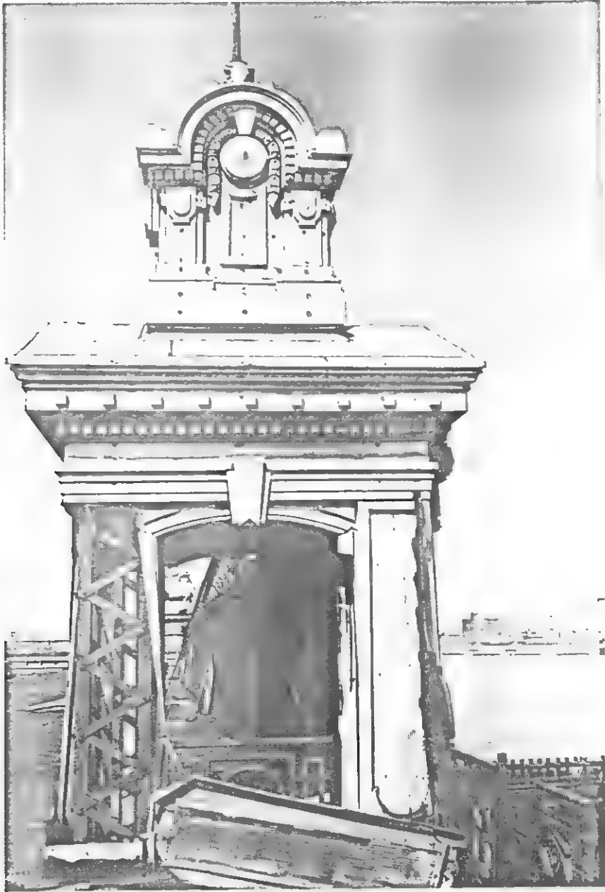
Northernmost belvedere of parapet over ferry slips.
